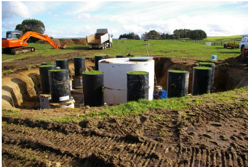
Figure 2 Lysimeter facility at Tihoi under construction.
